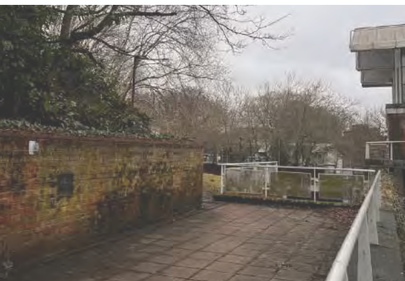
Significant level changes across the Carfax site re-inforced through retaining walls and steps, which limit level access routes.
